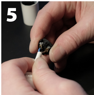
5 check connection with a steady pull
