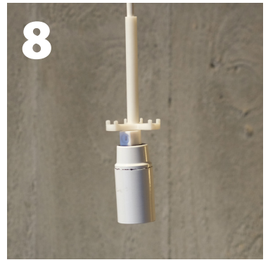
8 choose the right place for a pendant hook in the ceiling, hang the mount in the right height, cut the wire and connect it properly to electric outlet
